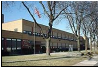
Brook Park Elementary School 30 th and Raymond LaGrange Park, IL 60526
